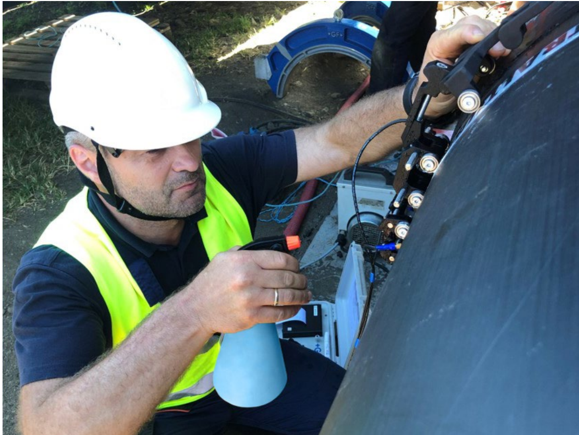
Non-destructive testing (Tahiti)
